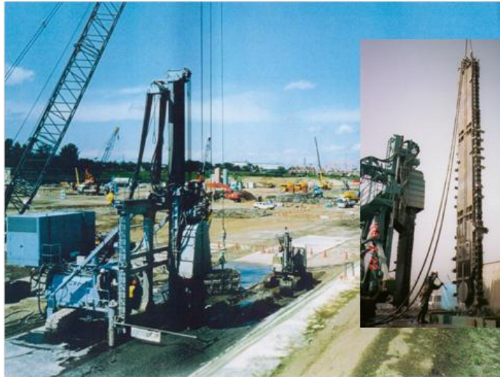
Photograph 6. TRD Method equipment.
