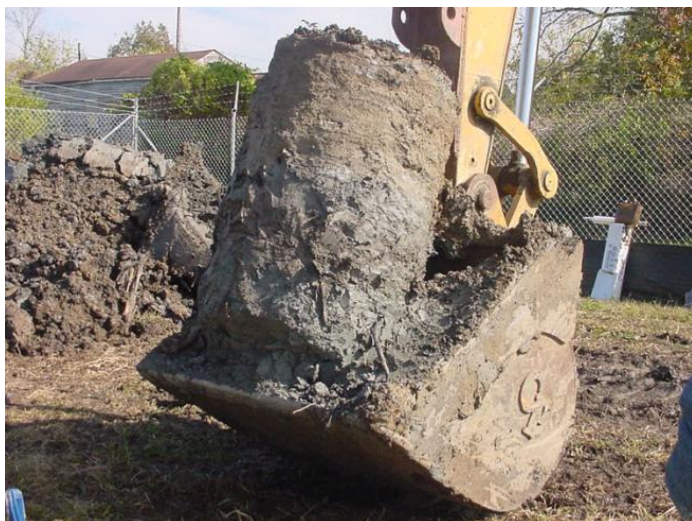
Photograph 1 . Excavated dry DMM test column, New Orleans, LA (Cali et al., 2005)
